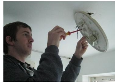
The new electric circuit and light are fitted.
