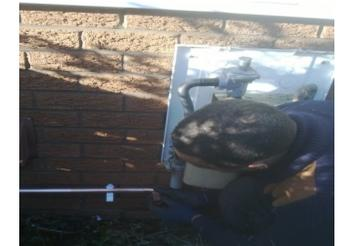
The new gas supply is run from the gas meter.
