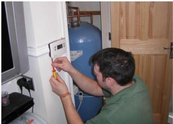
The electrician wires in the new programmer and thermostat.
