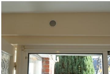
◀ The finishing off is completed which includes any builders work that is required. High level pipework is boxed in and painted to match your decoration.
